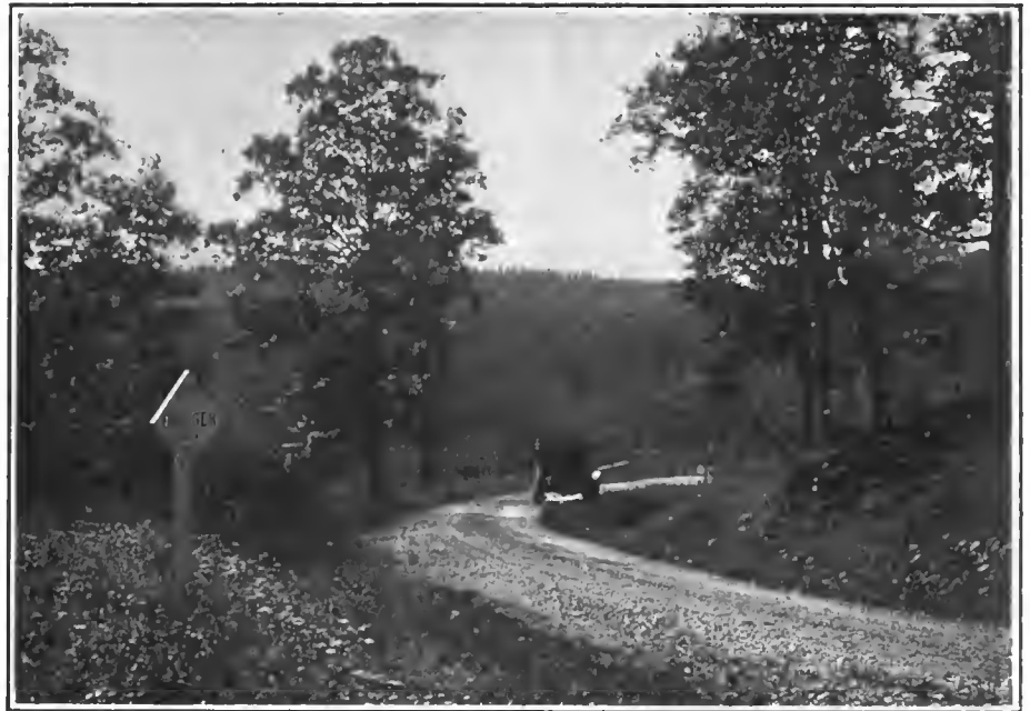
AN ALLEGHENY COUNTY ROAD SCENE SHOWING DANGER SIGN AT TOP OF HILL.
